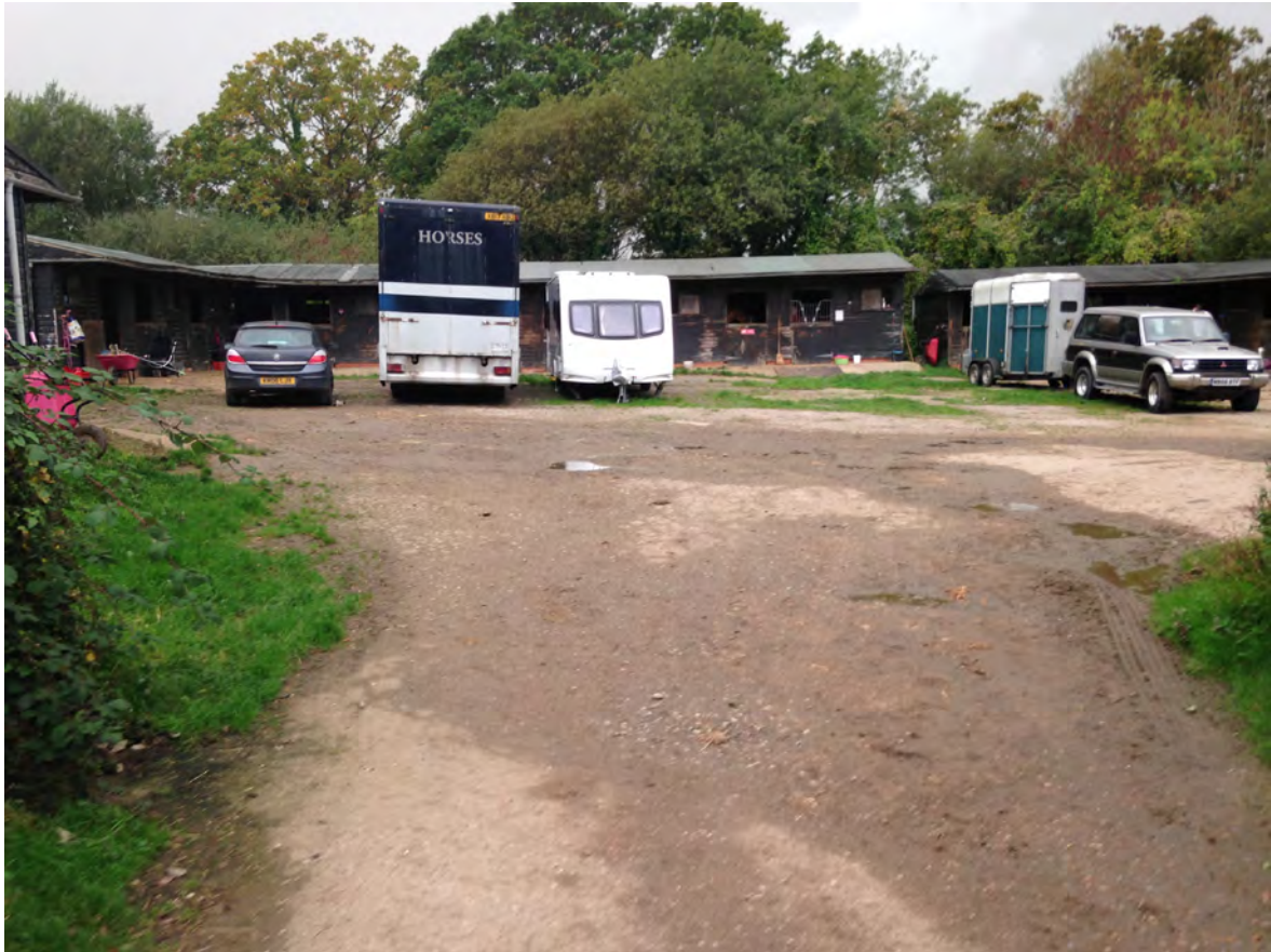
Plate 1: View of stable building in north central area of study site, facing west
